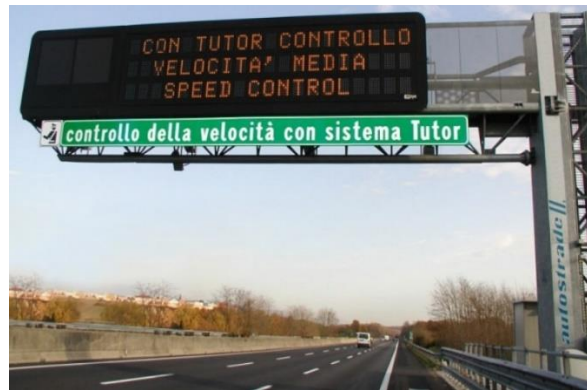
Figure 1: Beginning of the average speed control section by the "Tutor" system on the motorway in Italy.
