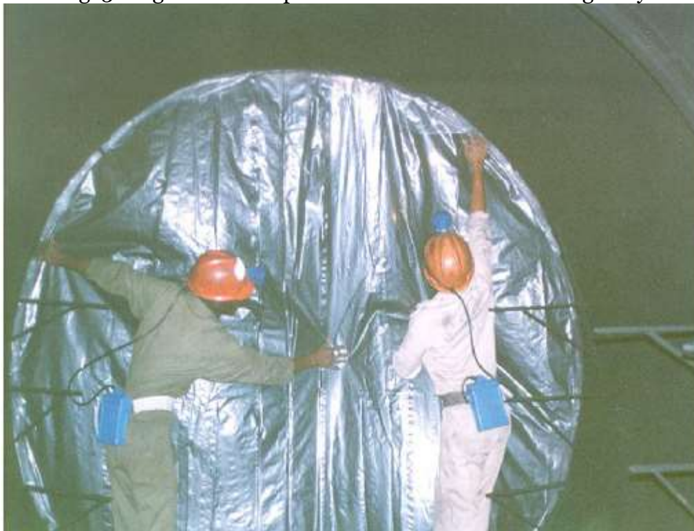
Fig. 4 Photograph showing the plastic membrane enclosing the methane chamber.
