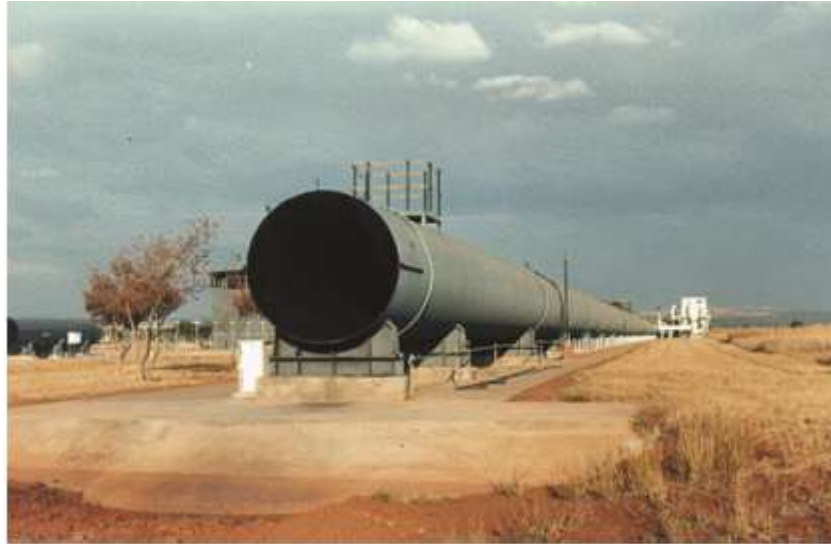
Fig. 2 Photograph of the 200 m test tunnel barrel and mouth
