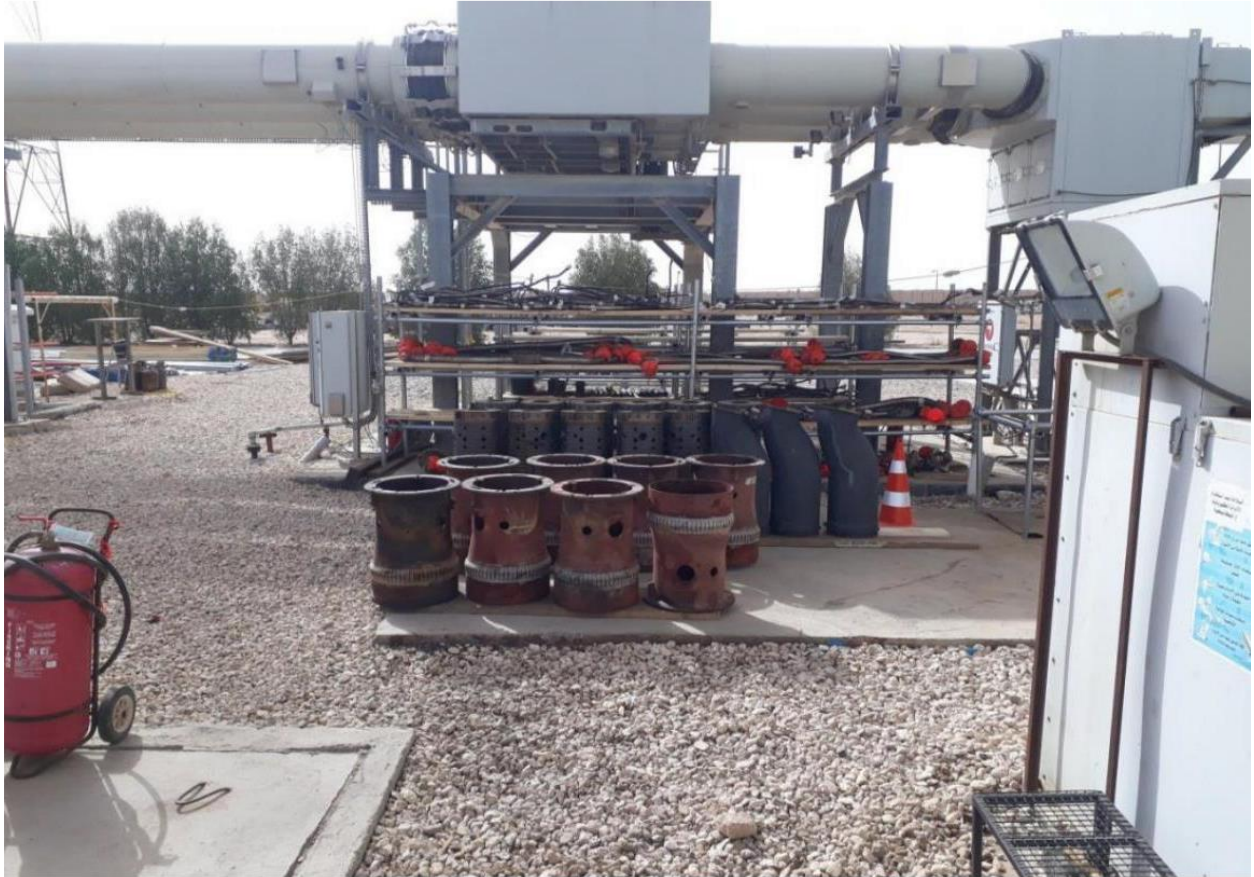
Figure 3 Dismantled old CI parts
