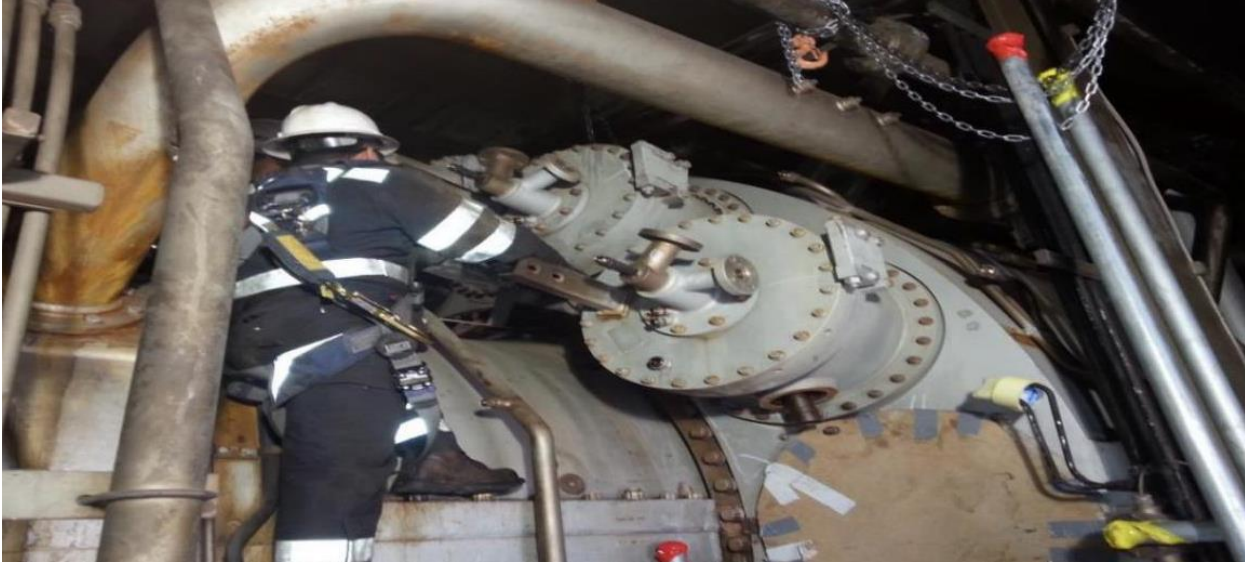
Figure 12 Closing the combustion chamber gates and installing fuel nozzles
