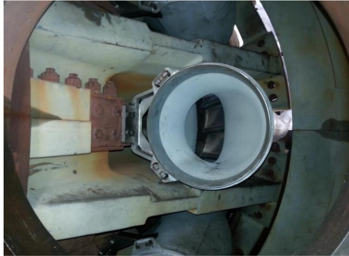
Figure 11 shows the installation of the new parts (N HOR BULL&TP)
