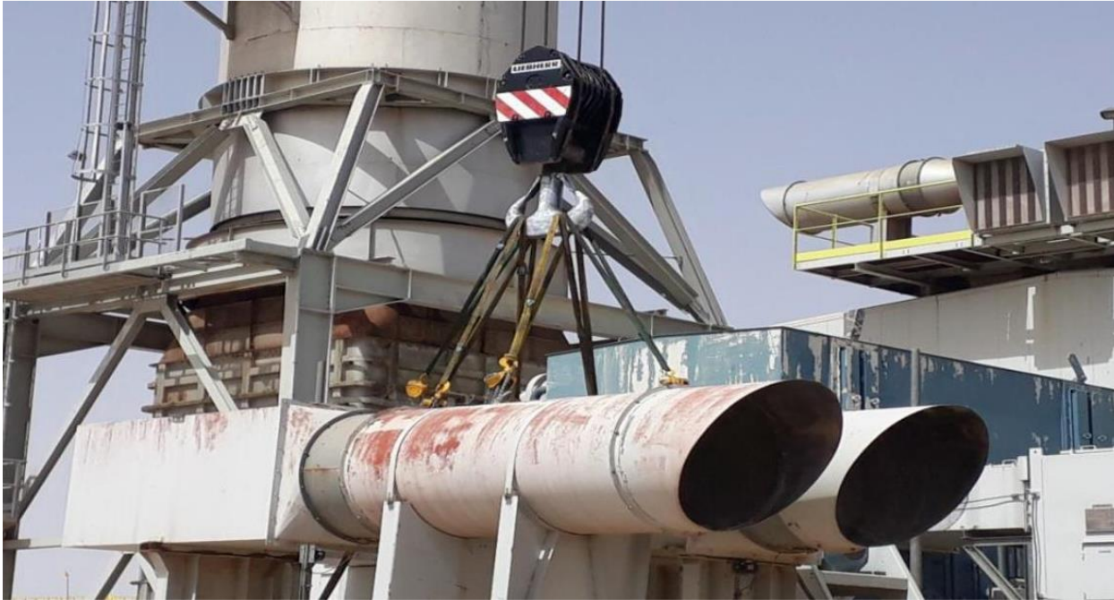
Figure 14 Reinstalling BT fans with air ducts
